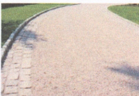
block curb and apron
